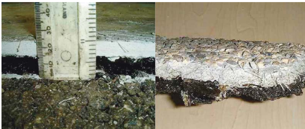
Figure 5.38. Delamination of the dense bitumen macadam below the edges HPCM pad
