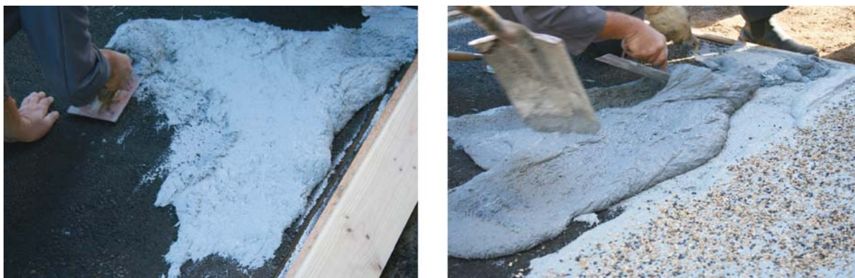
Figure 5.15. View of batches 1 (left) and 2 being spread immediately after mixing was completed
