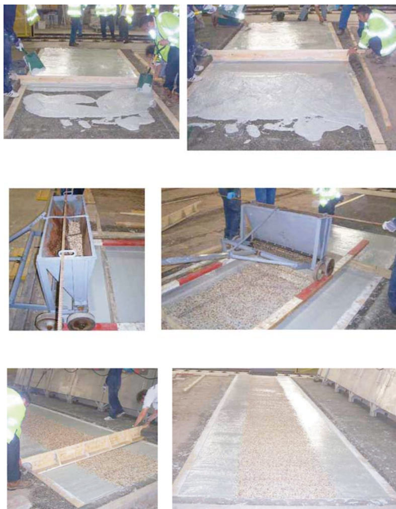
Figure 5.36. Construction of the HPCM test pad
