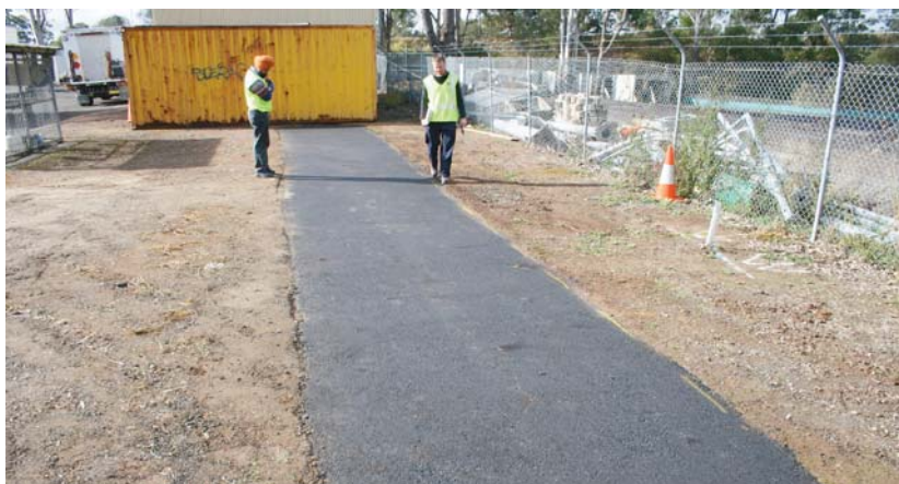
Figure 5.14. View of test site at RTA's St Marys work depot with the completed asphalt trial pad
