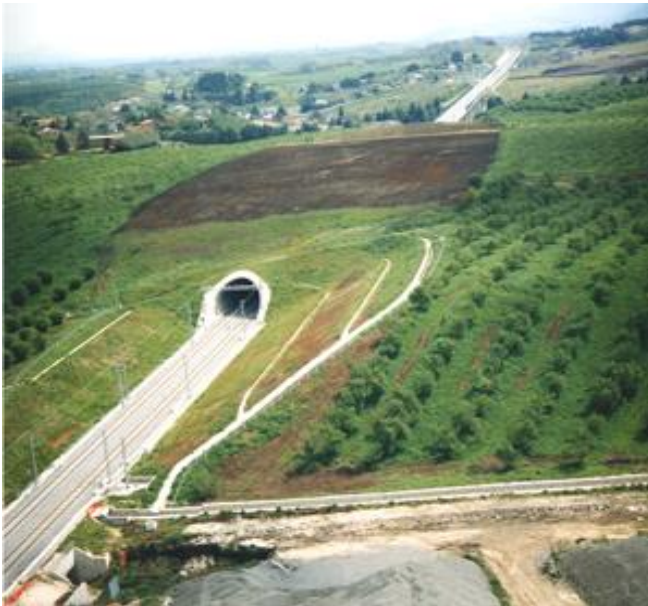
The Gelsi tunnel
