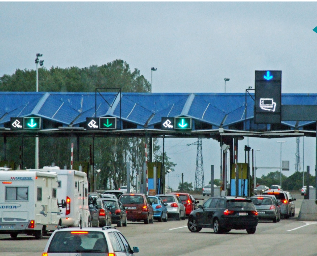
Tolling Station, near Paris, France
