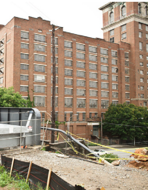
Construction work for the Atlanta BeltLine
