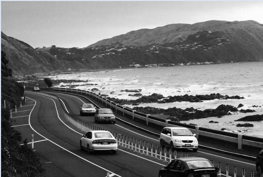
Figure 5.12. Rope-wire median barrier on the Centennial Highway, New Zealand
