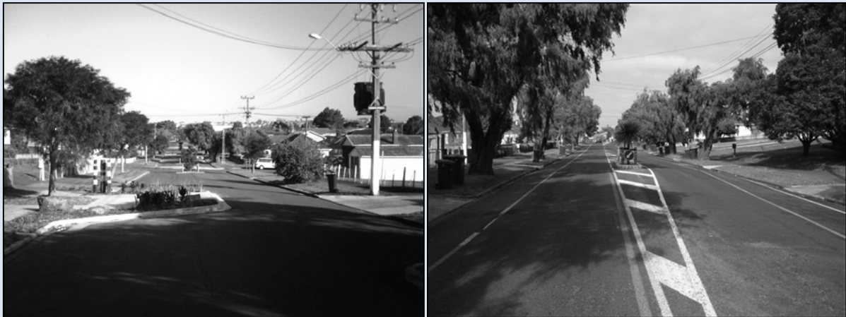
Left, Local road; Right, Collector road.
