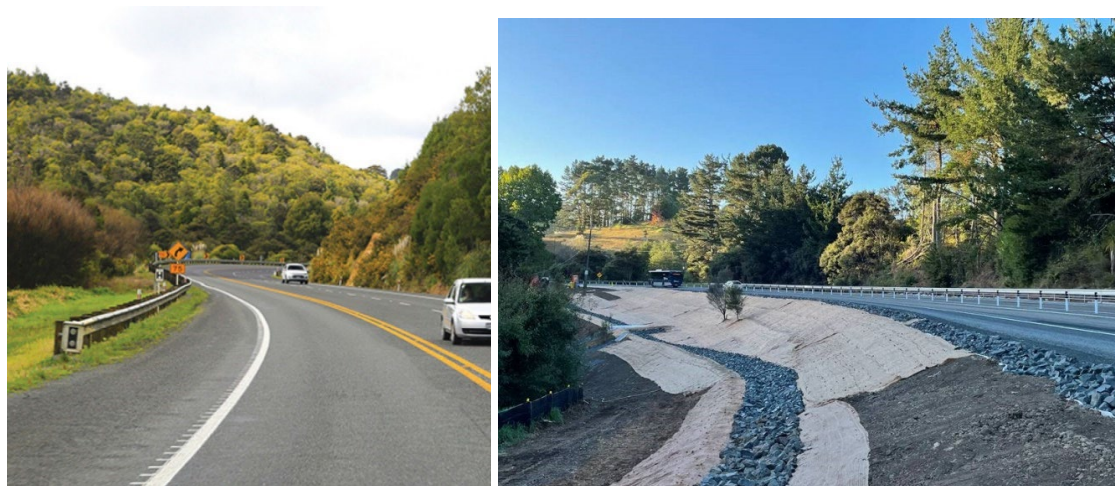
Figure 1. State Highway 1 Dome Valley before and during safety improvements
