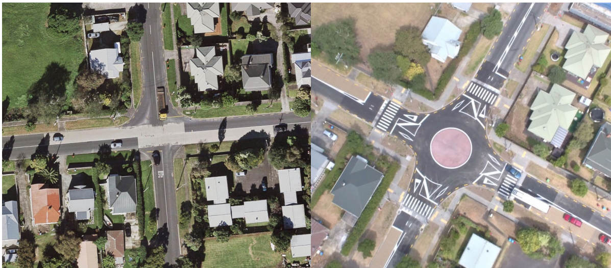
Figure 2. Church Street/Victoria Street intersection before and after safety improvements
