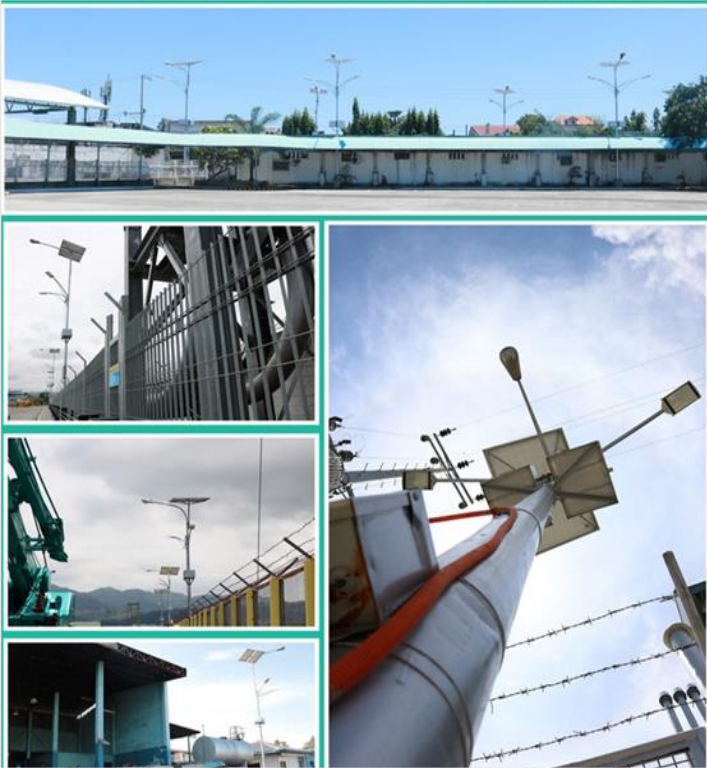
Installation of Solar powered port lighting
