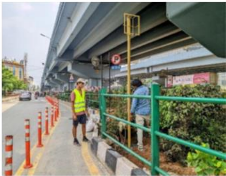
Installation of Bicycle Counter
