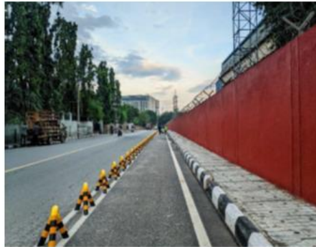
Installation of safe cycling infrastructure - segregated cycling lane
