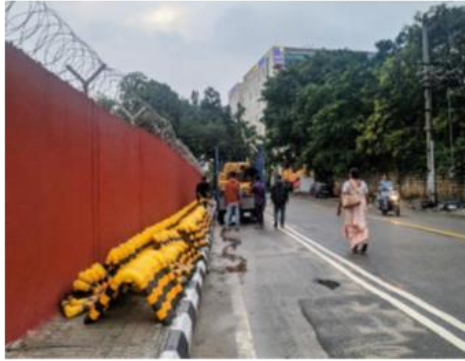
Installation of safe cycling infrastructure - segregated cycling lane
